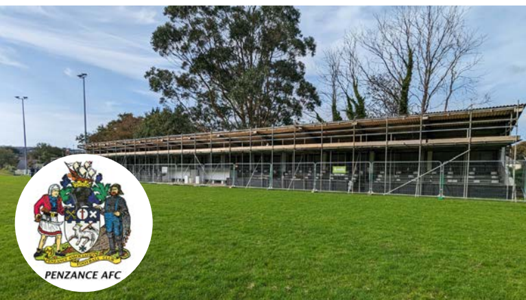
Start of the replacement roof works at Penzance Football Club - October 2023
